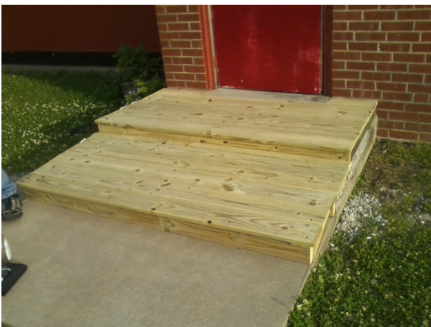
New Step covers added to the north door main entrance . . . . .
